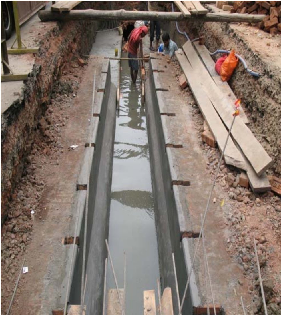
Sewer before top slab casting
