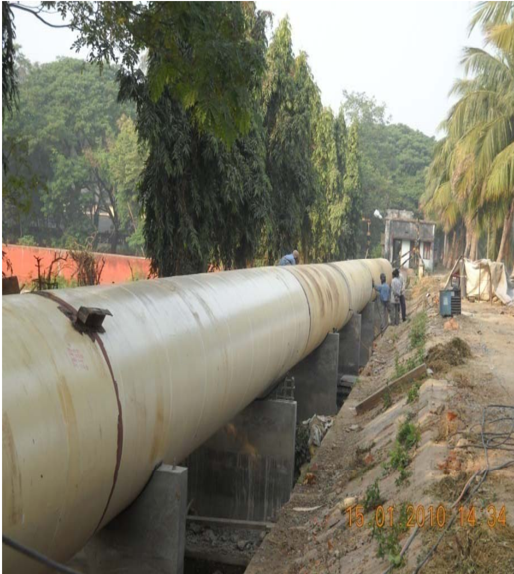
Pipes laid on raised pedestal
