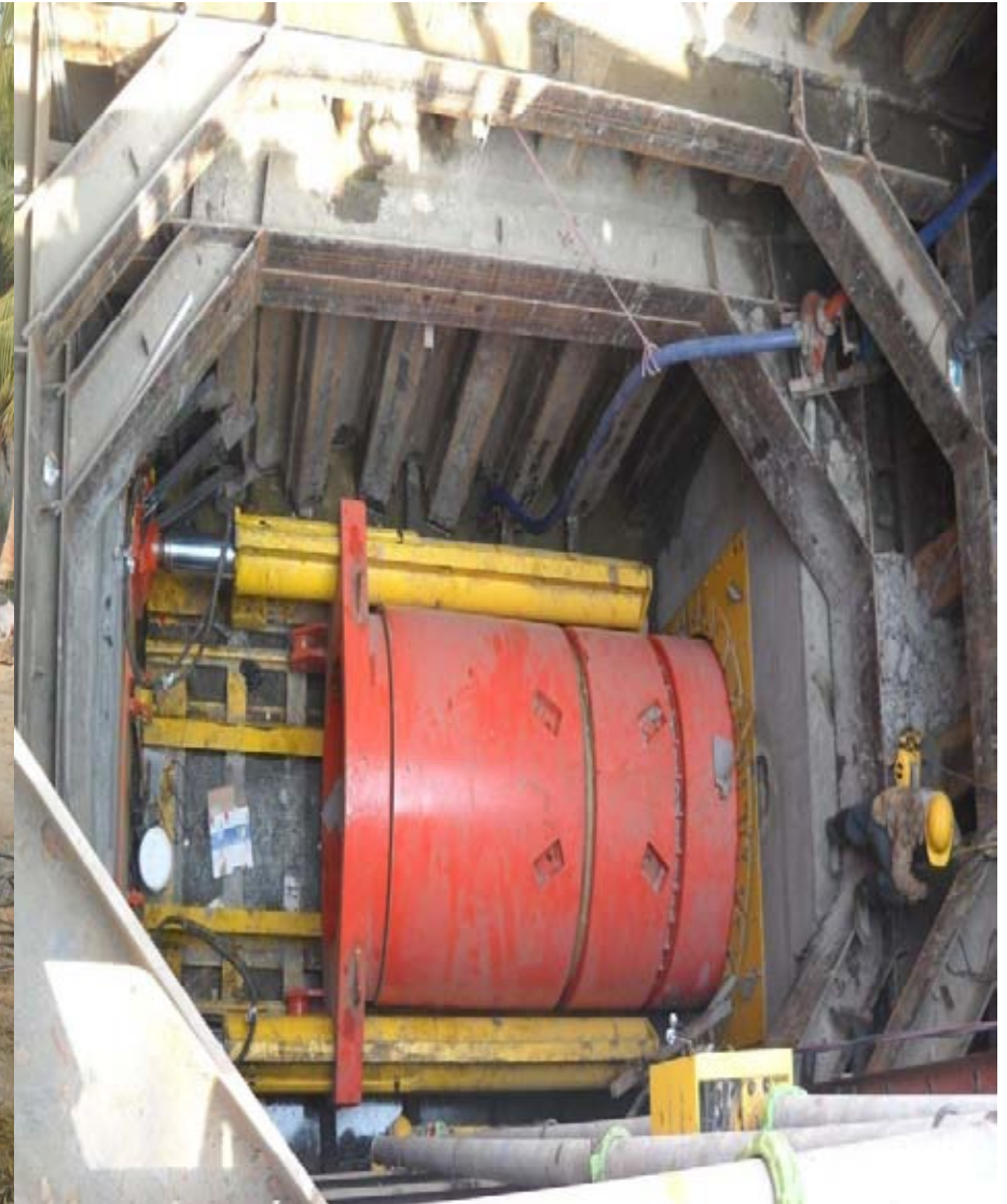
Pushing of Pipes through TBM
