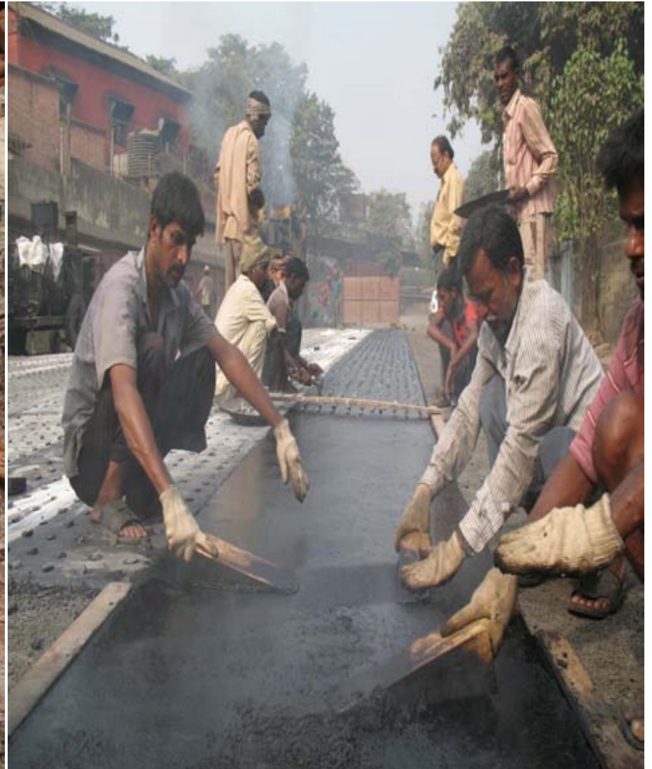
Mastic work is in progress after rehabilitation of sewer
